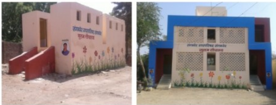
Sangamner: Newly constructed community toilets
