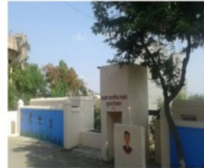
Sangamner: Newly constructed community toilets
