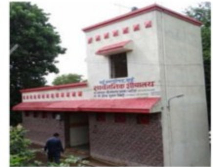
Well maintained CTs in Wai
