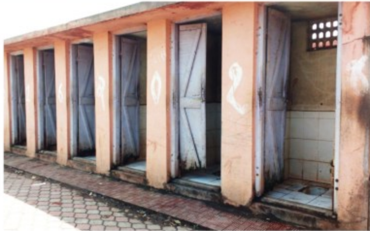
Reviewing the condition of existing CTs- Phaltan MCI
