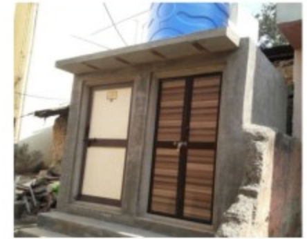
Wai: Completed Group Toilet in Wai
