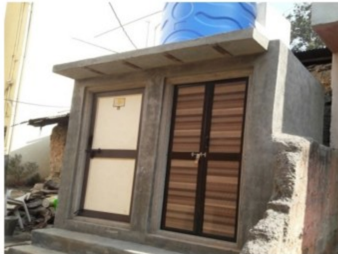
Wai - Completed Group Toilet
