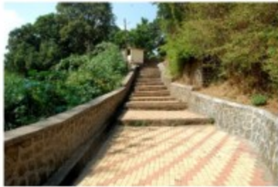
Malkapur: OD spot paved and community toilet constructed
