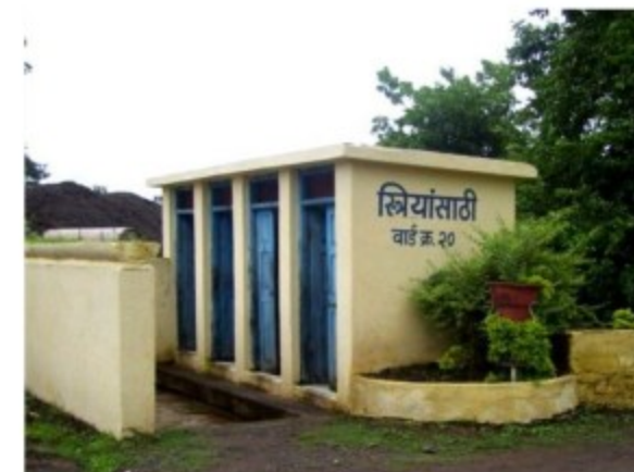
Special consideration for Women toilets
