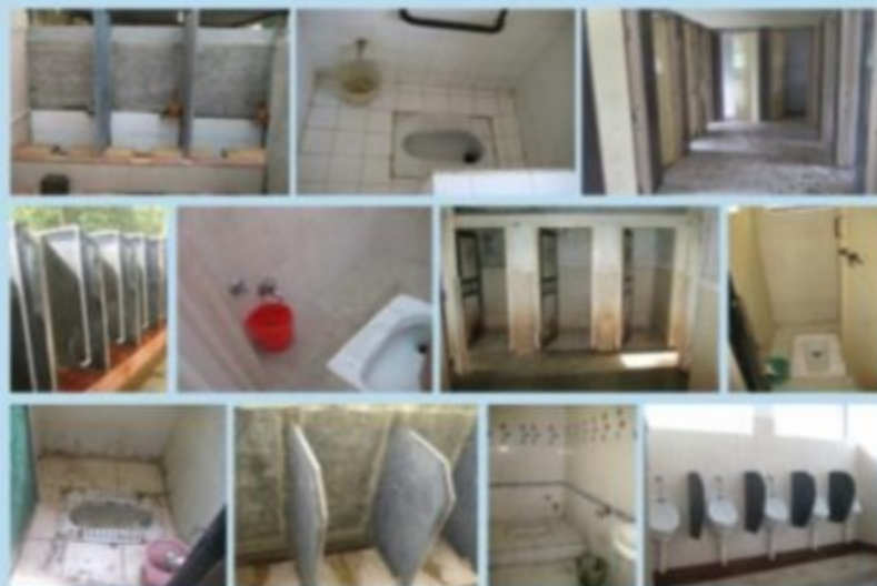
Condition of Toilets in Private Schools
